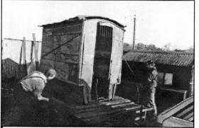
the fitting of a corrugated iron roof at some point during its enforced retirement. Unfortunately the wheels and the undercarriage were missing. Replacement wheels, axle, springs and shafts were all sourced locally. The vehicle was repainted and embossed with a royal coat of arms to complete its restoration. It was then kept at the jail as an exhibit being taken to various functions in and around Aberdeen. In 1991 it took a central role in the Jail's centenary celebrations
